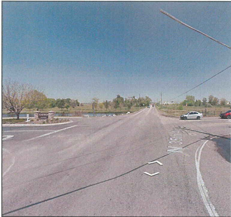
"C" Street Intersection Looking North
